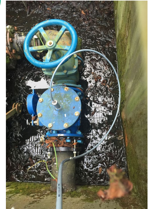
A sensor head in a non-return valve.
