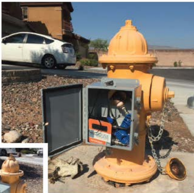
(top) A custom security box protects the Syrinix PIPE-MINDER units, allowing them to be left in place as needed.
