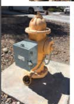
(top) A custom security box protects the Syrinix PIPE-MINDER units, allowing them to be left in place as needed.
