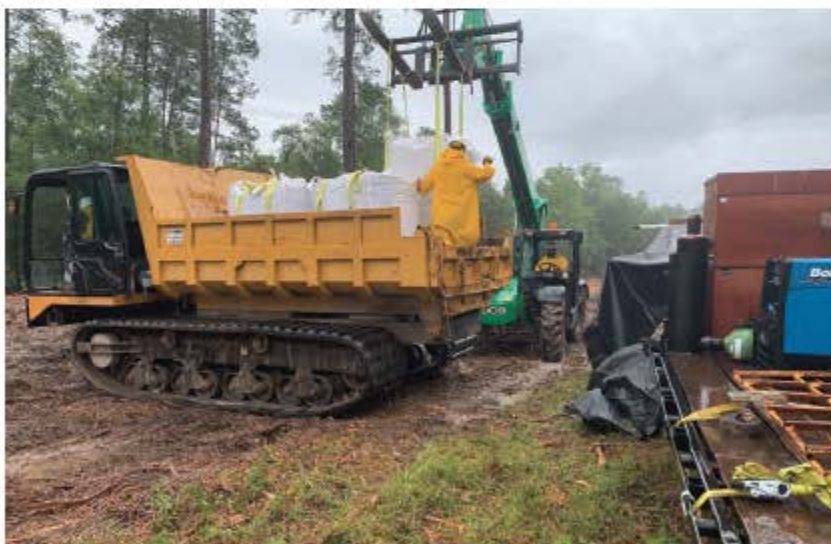
TerraFirma utilized the Marooka MST3000VD to move 3,000 lb. super sacks of specialty filter gravel and other materials from the staging area to the drill pad.
