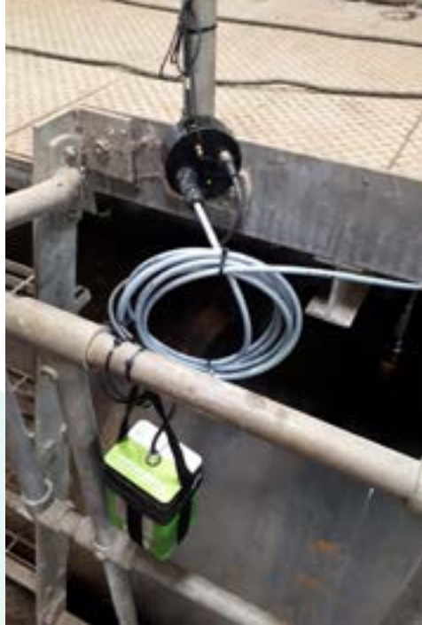
Left and centre: Installation of the Pipeminder sensors at Anglian Water.
